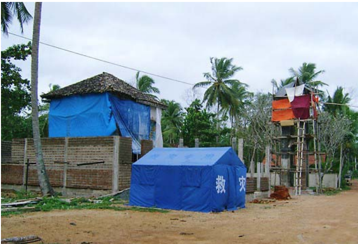
'Buddu ge' and bell tower under repair
